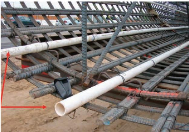
[FIG. 1] Typical Drilled Shaft Reinforcing Cage with PVC Sonic Access Tubes Added
