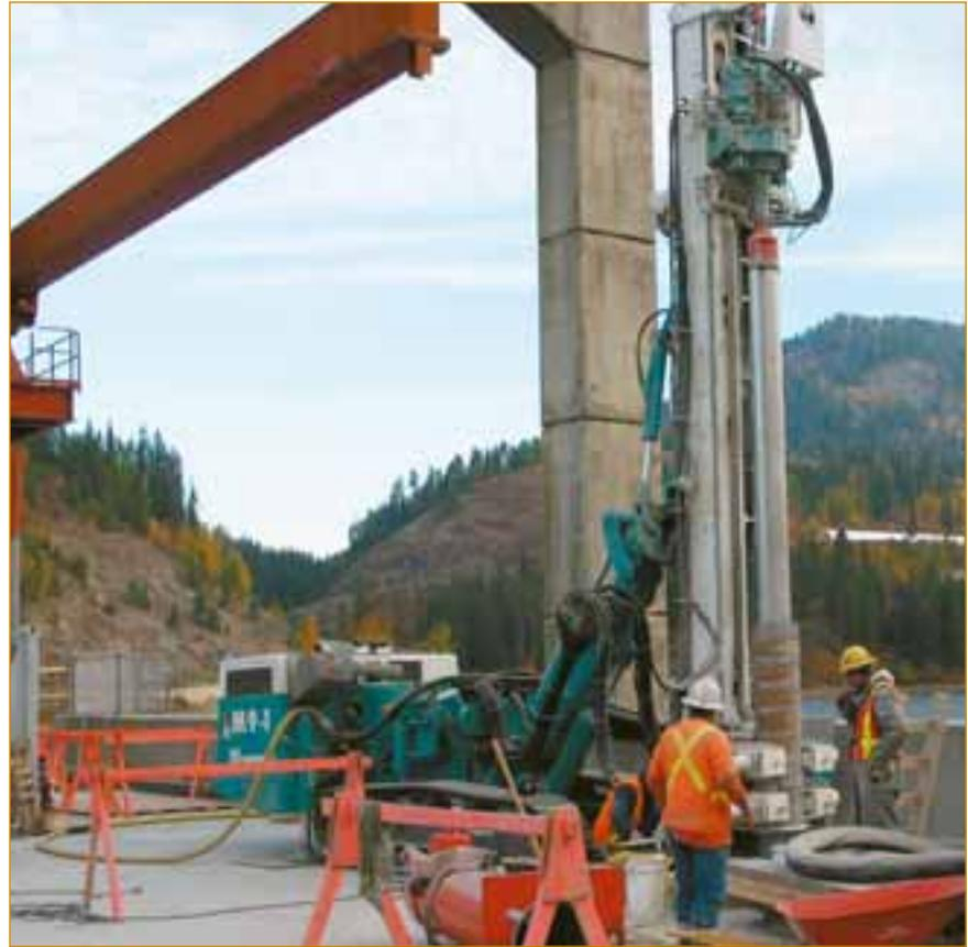
Figure 5, **Anchor Hole Drilling**
