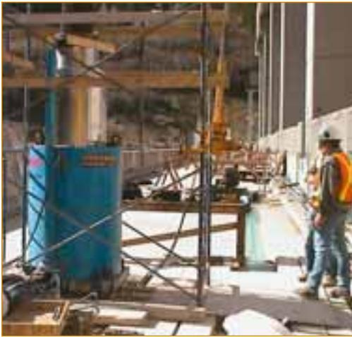
**Figure 8, Installation Jack System Stressing**
